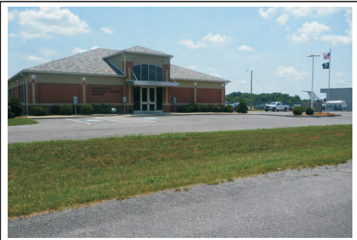
Photo 27: Hopkinsville-Christian County Airport terminal facility; facing south.
